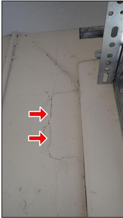
9.7 Item 1(Picture) Typical crack at garage wall
