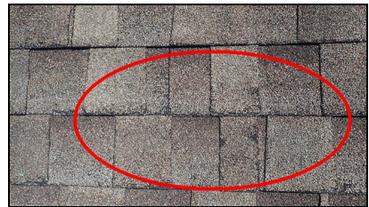
4.2 Item 3(Picture) Granular loss
