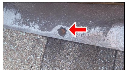
4.5 Item 3(Picture) Rusted vent nail
