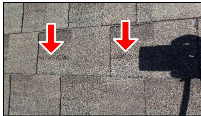
4.2 Item 2(Picture) Granular loss
