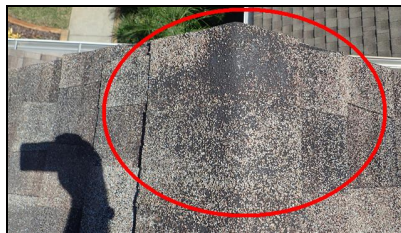
4.2 Item 5(Picture) Heavy granular loss at gable ridge
