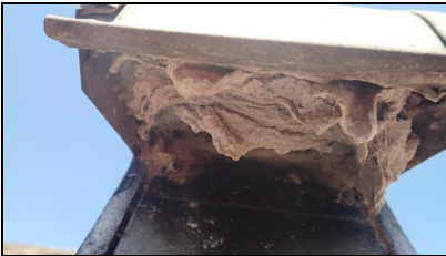
13.3 Item 1(Picture) Clean dryer vent hood
