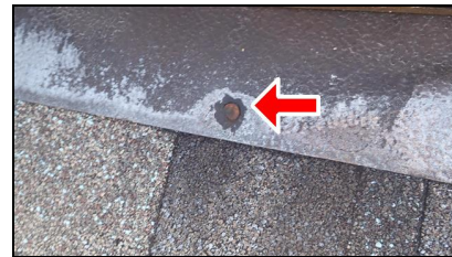
4.5 Item 3(Picture) Rusted vent nail
