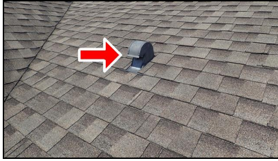
13.3 Item 2(Picture) Clean dryer vent hood
