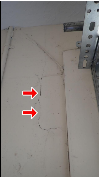
9.7 Item 1(Picture) Typical crack at garage wall
