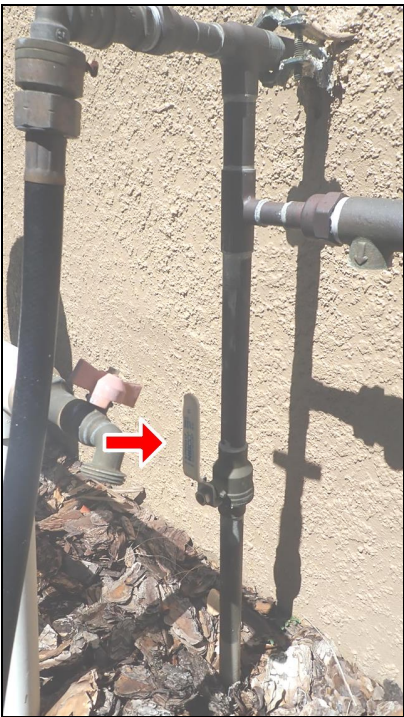
5.2 Item 1(Picture) Main water supply shut off valve
