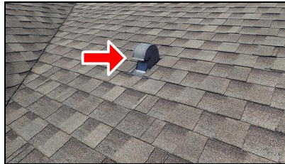
13.3 Item 2(Picture) Clean dryer vent hood
