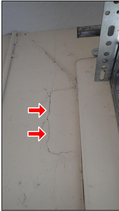
9.7 Item 1(Picture) Typical crack at garage wall
