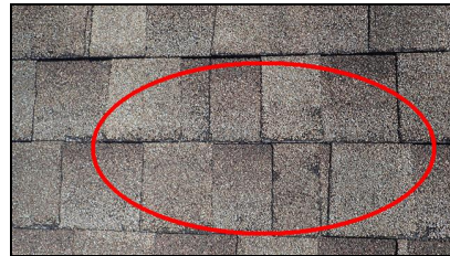
4.2 Item 3(Picture) Granular loss
