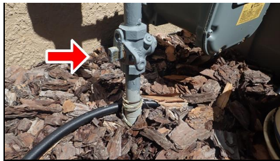
5.11 Item 2(Picture) Gas meter shut off valve
