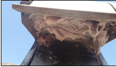
13.3 Item 1(Picture) Clean dryer vent hood
