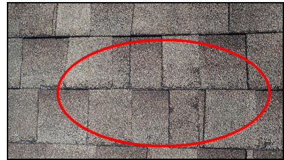
4.2 Item 3(Picture) Granular loss
